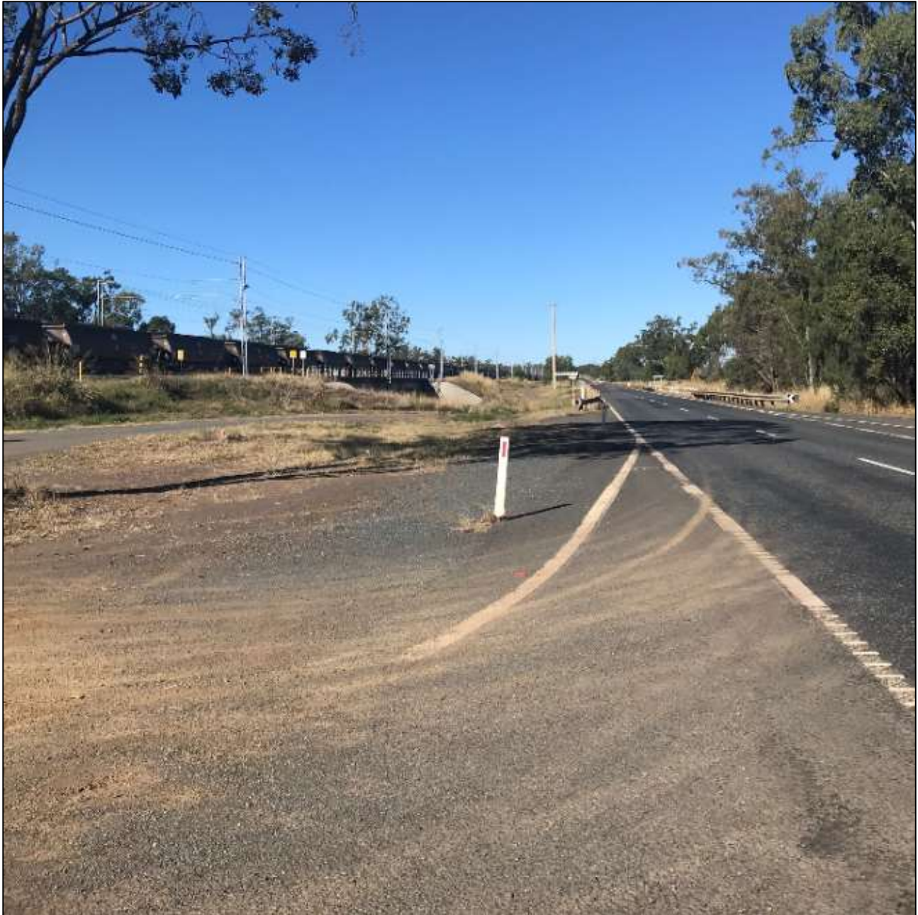
Figure 3-5 Capricorn Highway / Red Hill Road (facing east)
